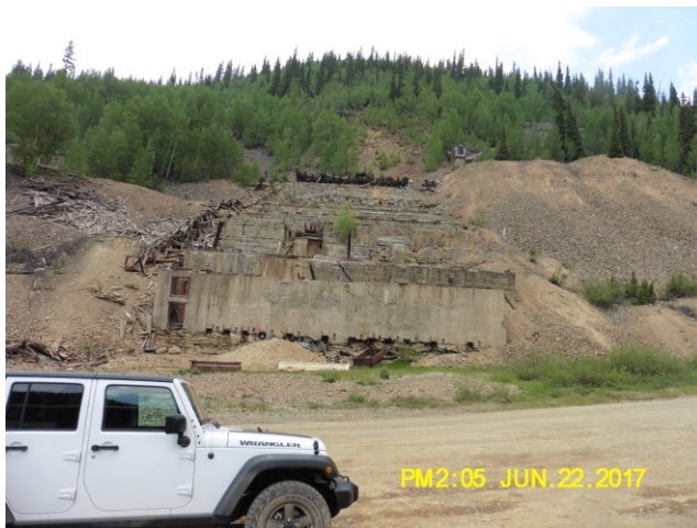
Mill foundations and waste rock piles Gladstone, Silverton CO
