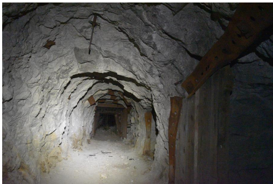
FIGURE 88. Looking north down the Wind Mountain nepheline syenite adit. The back (top) is approximately 10-15 ft high.
