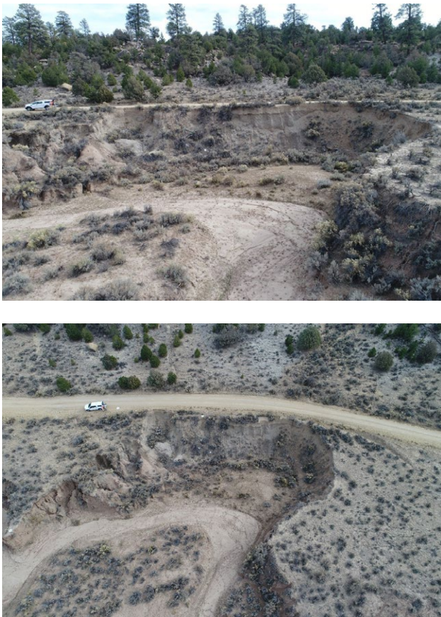
Figure 7.21. UAV photographs of cutbank erosion threatening infrastructure in Tapicito Creek approximately 500 m downstream of New Mexico Highway 537. Top photograph shows Tapicito Creek (in bottom left and center, flow direction from left to right) and 6-m-tall cutbank. Note position of road atop cutbank. Photo taken from approximately the same elevation as the road. Bottom photograph shows same location from an altitude of approximately 50 m.
