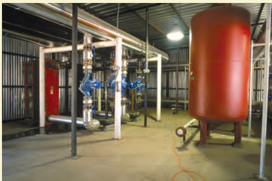
Heat exchangers, pumps, and tank at Masson Radium Springs Farm geothermal greenhouses. Heat exchangers are used to transfer heat from geothermal water to a closed-loop fresh water heating system.
