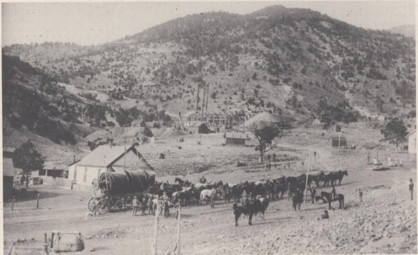
Brown's great discovery at Kelly mine, southwest of Socorro, was that massive amounts of dry-bone ore (valuable smithsonite) were masquerading as limestone. This led to major investment and development in the area as depicted in this photo, where a large, double-drum hoist is being delivered to the future Taylor Shaft site at Kelly (ca. 1907, NMBM&MR photo collection #1505).
