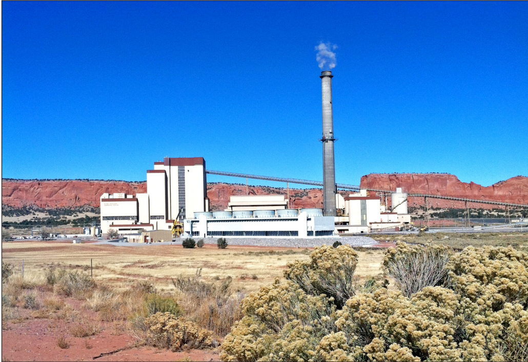
Escalante Generating Station. Photo courtesy of Tri-State Generating and Transmission Association.
