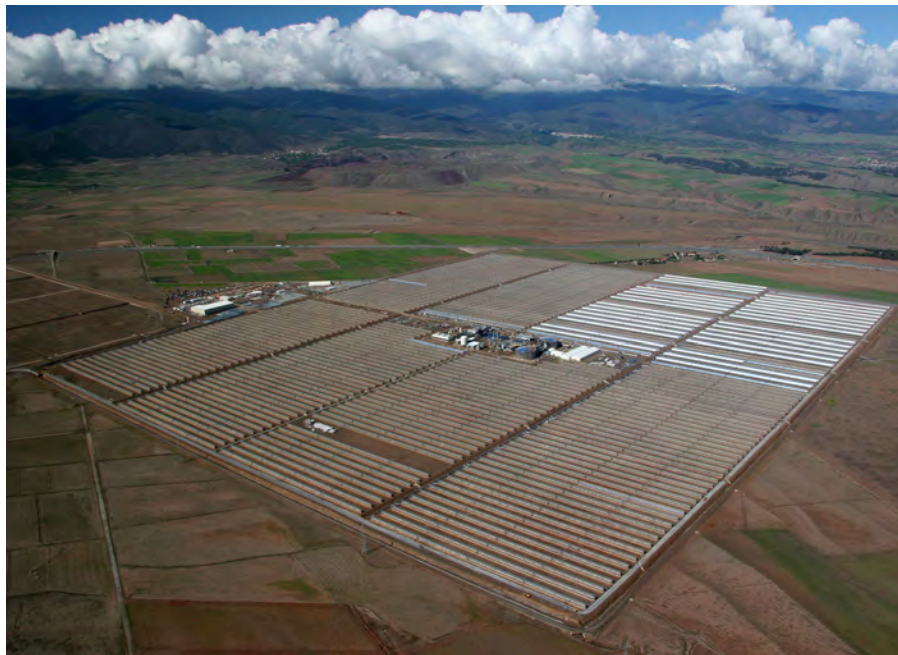
Spain has become a leader in solar energy, although this industry is now troubled due to unsustainable government financial subsidies. The 150 MW Andasol solar power station, shown above, is a commercial parabolic trough solar thermal power plant, located in southern Spain. The Andasol plant uses tanks of molten salt to store solar energy so that it can continue generating electricity even when the sun isn't shining. This photo shows the first phase only; the facility is now three times this size. Source: en.wikipedia.org/wiki/Renewable_energy_commercialization#mediaviewer/File:12-05-08_AS1.JPG . From Wikimedia Creative Commons.
