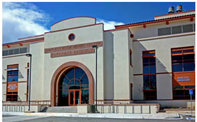
New Mexico Bureau of Geology's new building is located at the corner of Leroy Place and Bullock Street on the New Mexico Tech campus. The Mineral Museum is on the right and the Publication Sales office is on the left of the front main entrance. Photo by Leo Gabaldon.
