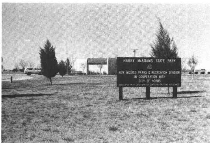
FIGURE 1—Looking northeast at the visitor's center with the park in the background.
