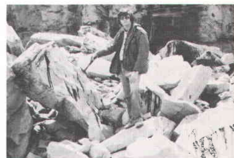
FIGURE 2—BROKEN, WEATHERED SANDSTONE SHOWING BLEEDING ASPHALT.
