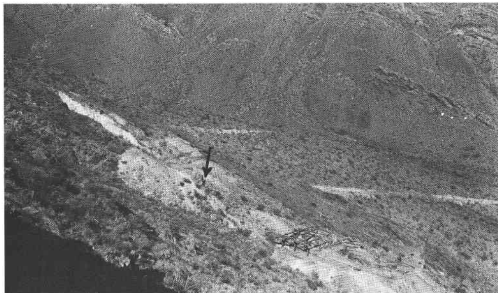
FIGURE 1—VIEW NORTHEAST OF MAIN WORKINGS, Red Rock talc claim. Framework of sorting shed in foreground; arrow indicates marker at southeast end line of claim.
