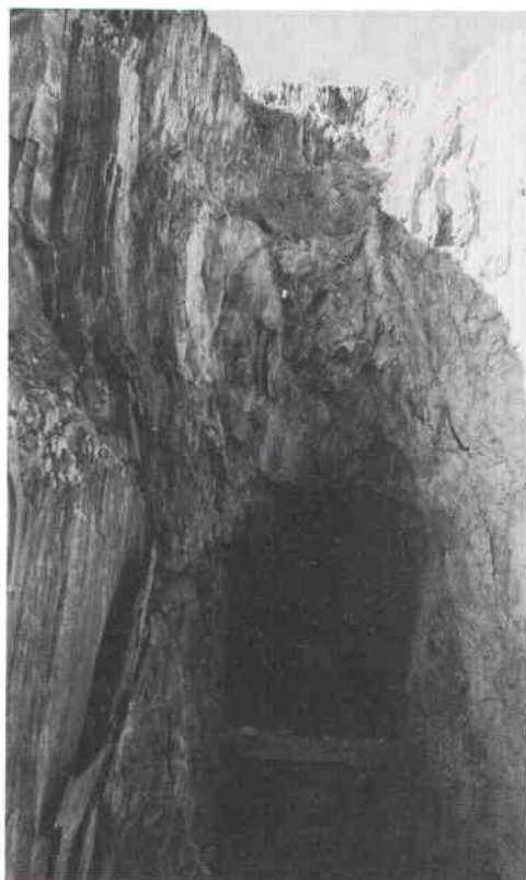
FIGURE 6—VIEW NORTHWEST INTO OPEN CUT AND INCLINE TO STOPE SHOWING mine stalls in place and talc in face of cut.
