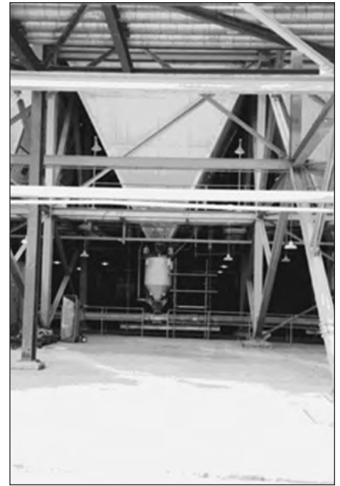
FIGURE 3—Ash hopper at the bottom of an electrostatic precipitator and ash conveying line. Coronado Generating Station, St. Johns, Arizona.
