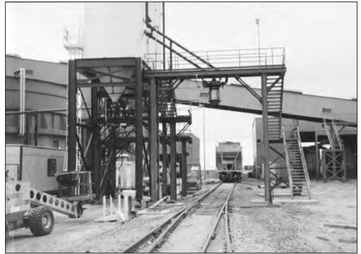
FIGURE 10—Mineral Resources Technology load-out facility at Coronado Generating Station, St. Johns, Arizona.
