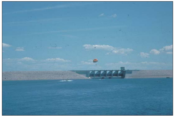
FIGURE 4—Brantley Dam, looking south across the lake. Photo courtesy of New Mexico State Parks.
