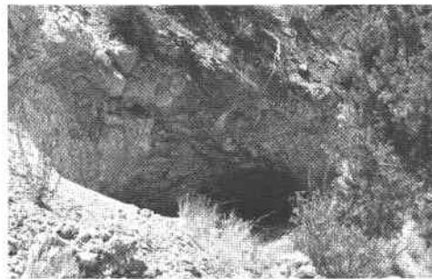
FIGURE 6—THE UPPER ADIT AT THE SALINAS MINE; opening is about 4 ft high, with a 3-ft thickness of barite above.
