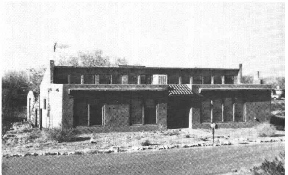
FIGURE 1—South-facing home in Socorro, New Mexico, with exterior, lightweight, conventional insulation covering adobe walls. Winter heating is provided by windows on upper level and fireplace on southeast (right) corner of home.
