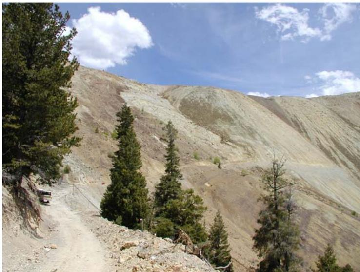
Figure 5. Access road cut across the Goathill North rock pile.
