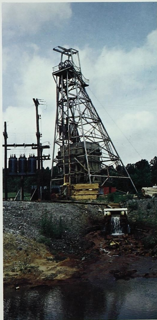
Headframe over the underground tungsten mine which is being evaluated by the Company.
