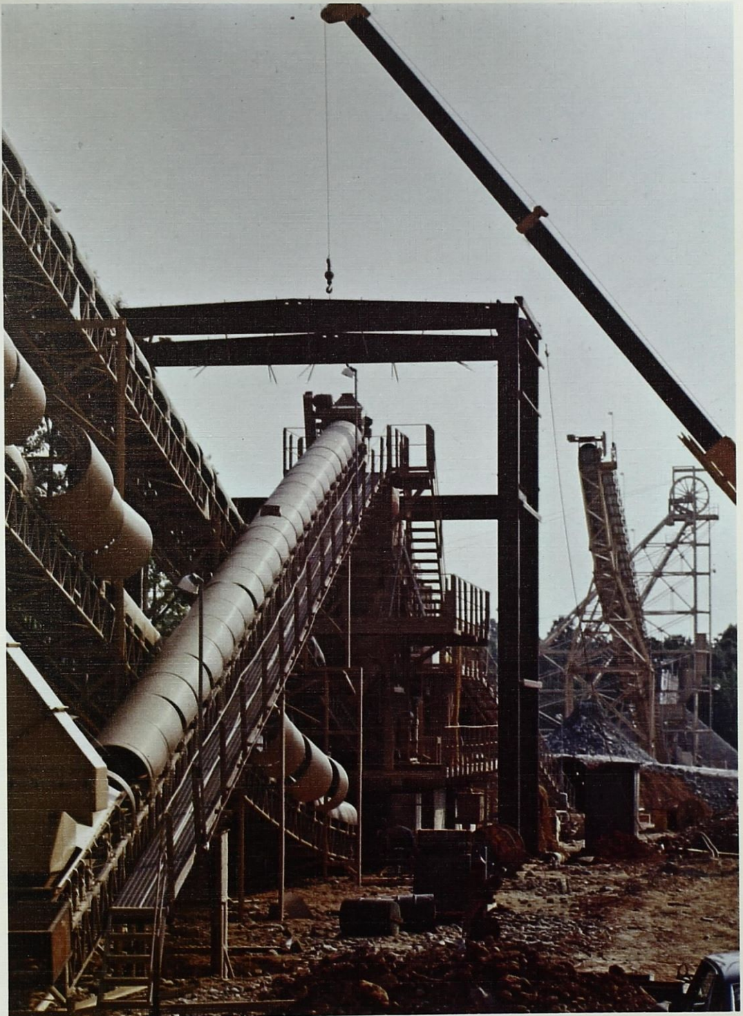
Constructing tungsten ore conveyor and crushers
