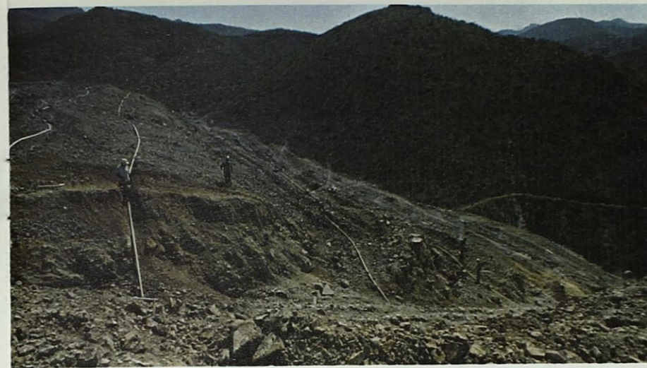
Acid and water are sprinkled on terraces (left); copper-bearing solution seeps from bottom of ore body (center) and flows down channel (below) to precipitation plant where cement copper (bottom center) is produced.
