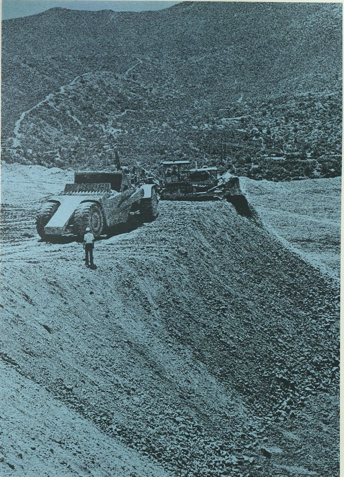
Building Leaching Heaps at the Bluebird Mine
