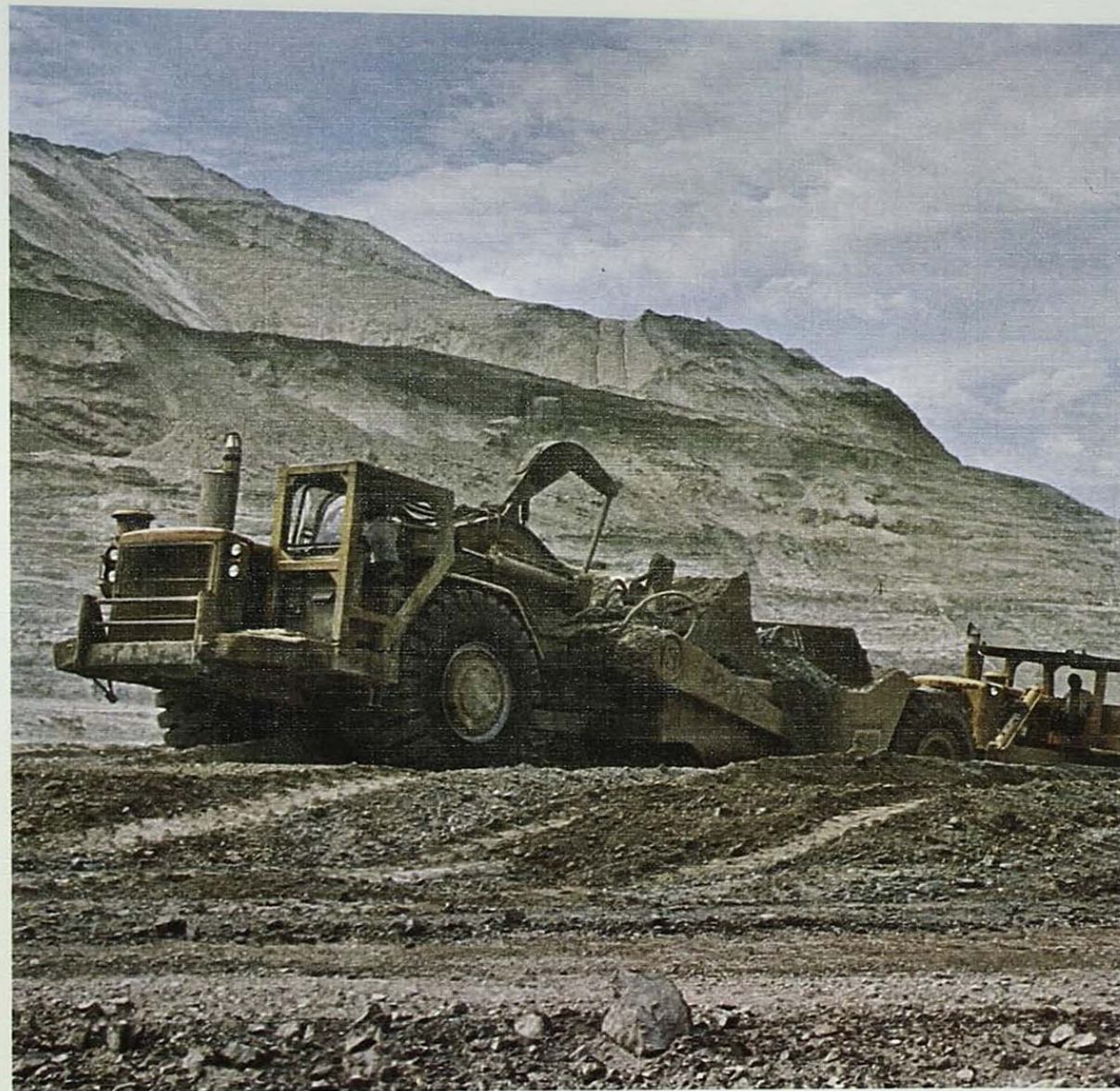
Loading Scrapers with Ore in Bluebird Pit
