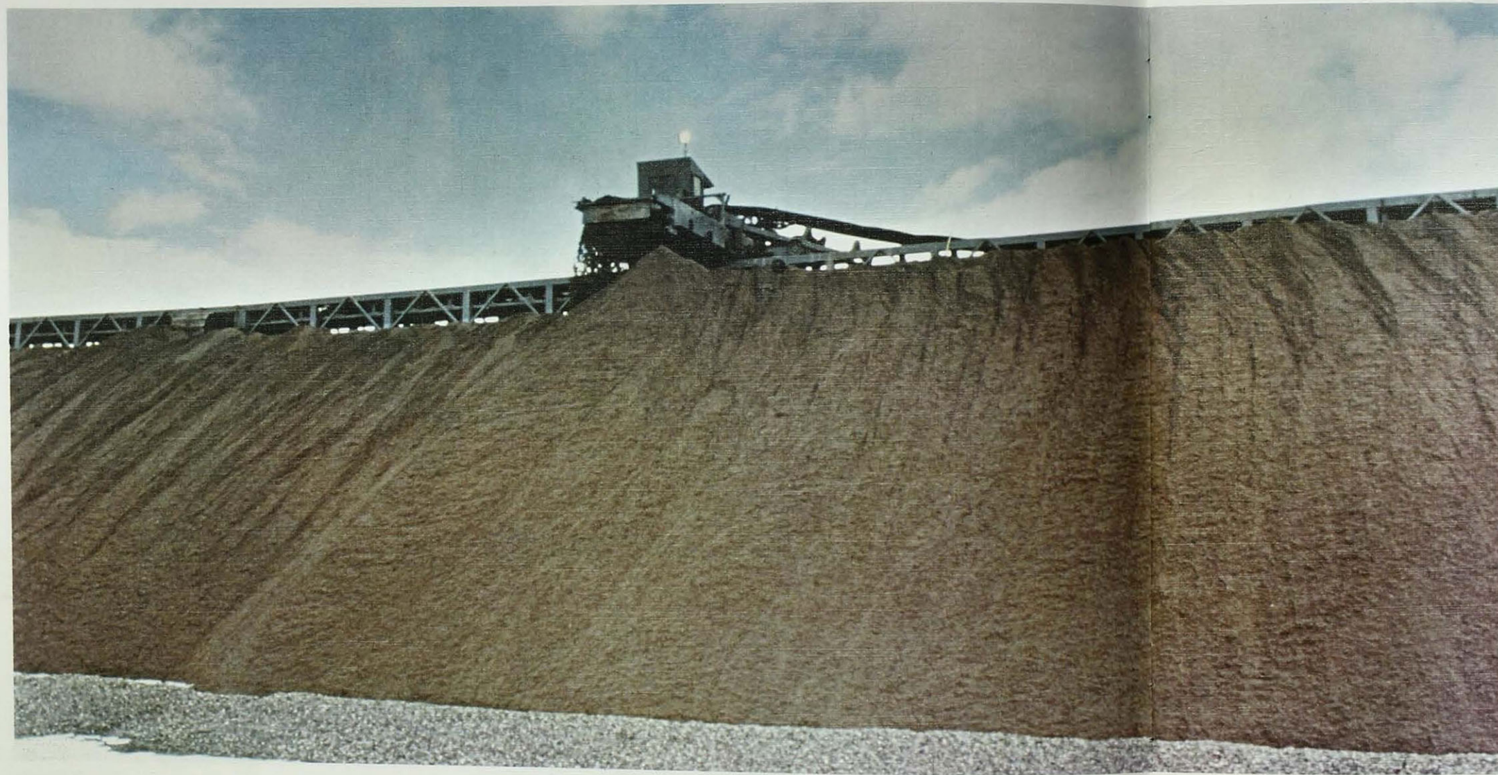
Spreader-Conveyor in Operation
