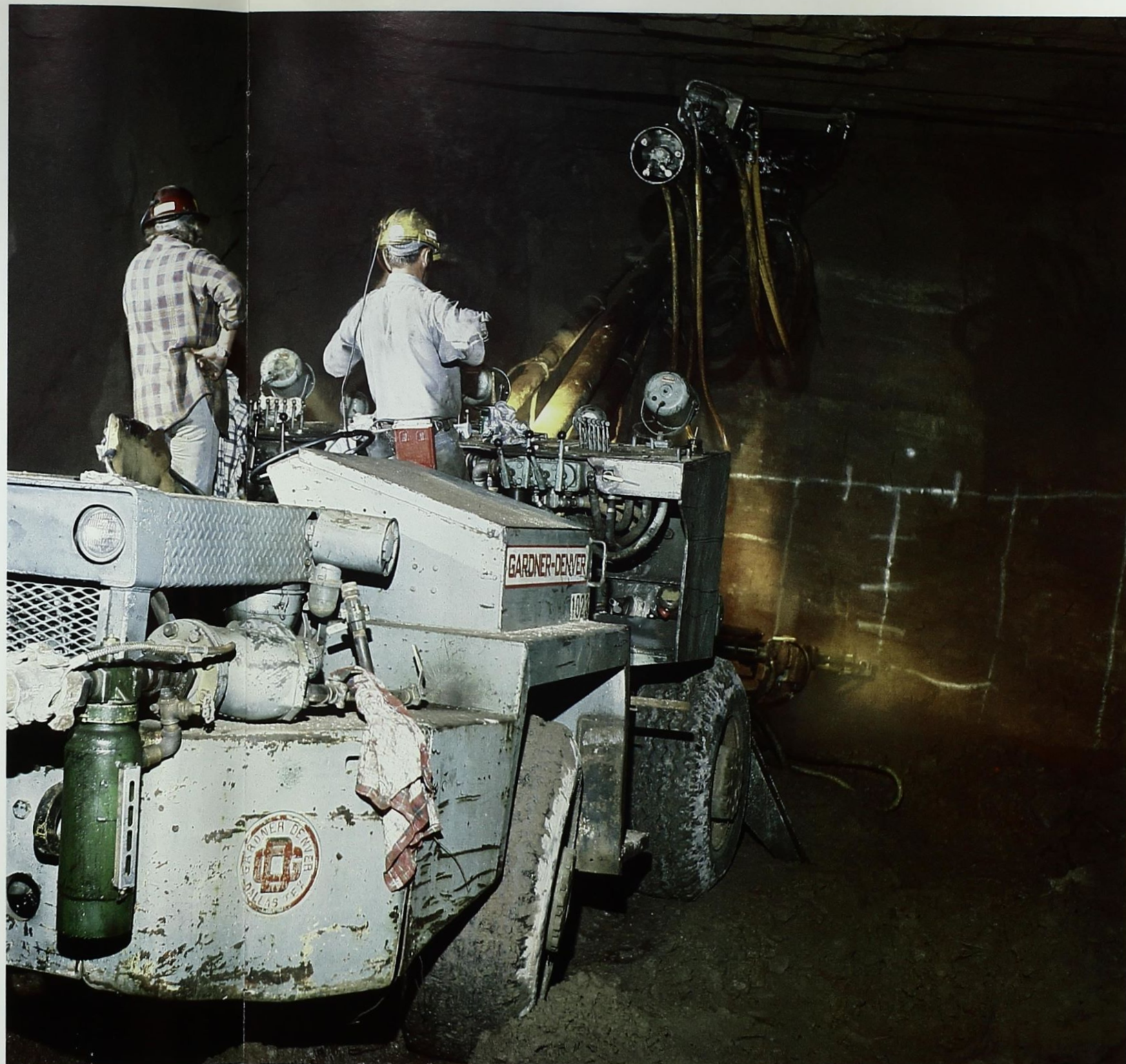
Drilling Blast Holes in Decline at the Escalante Mine.
