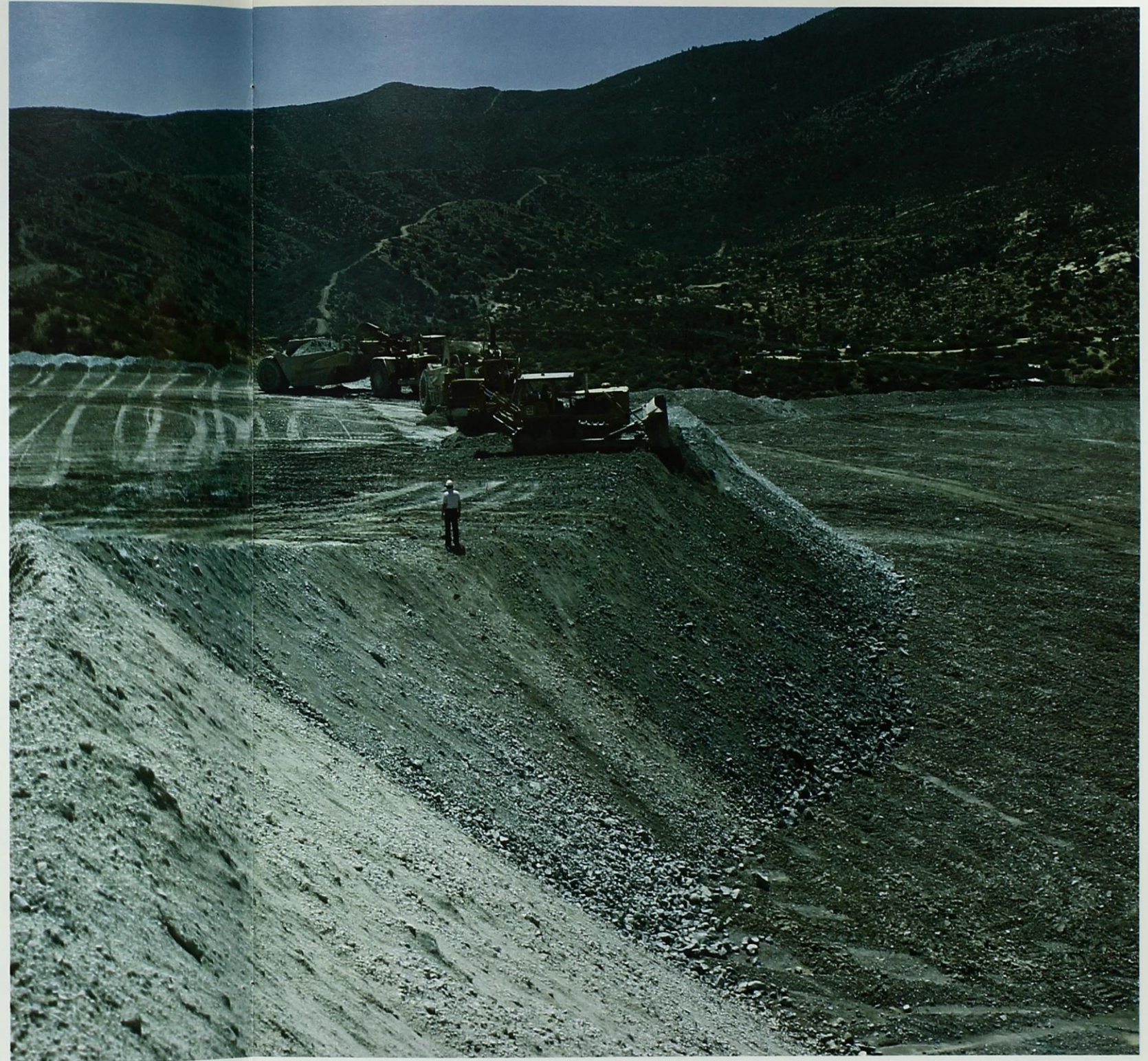
Heap Construction at Bluebird Mine
