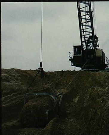
Stripping overburden from clay deposit with dragline
